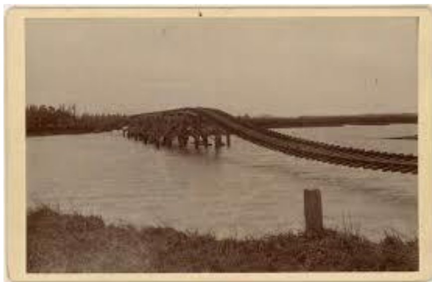
Creator unknown: Photograph of the flood damaged Waitangi railway bridge at Clive. Ref: PAColl-8256. Alexander Turnbull Library, Wellington, New Zealand. /records/23071786
